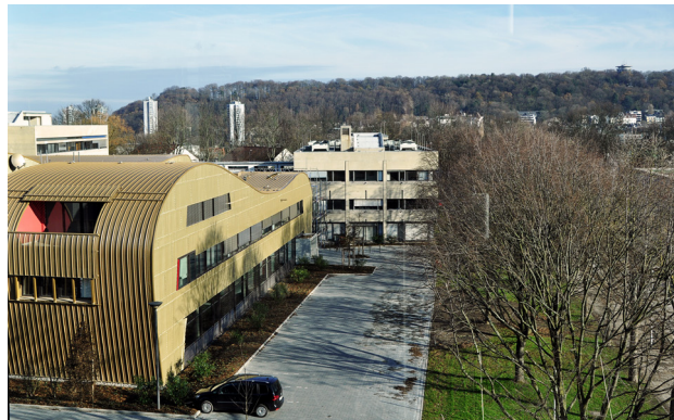
Main building of the IT Center, Seffenter Weg 23, extension building on the left side, Kopernikusstraße 6.
