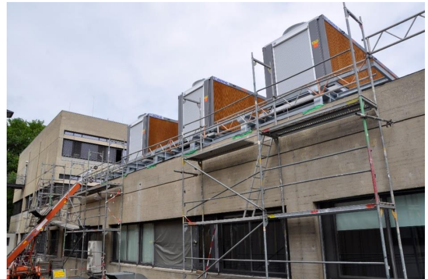
Cooling towers (construction phase)
